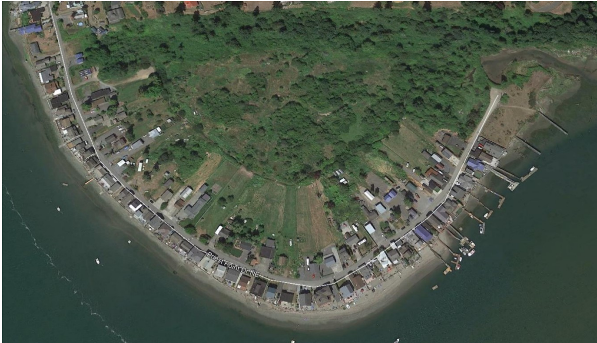
Figure 2. Priest Point is a “spit” formation created by the wind and wave induced movement of sand and gravel. The high elevation on the spit are naturally at the highest level of tides and storm surge. Houses built on the spit began as fishing shacks that were not of great concern. Fishing shacks upgraded to houses over time represent considerable investment that is at risk from sea level rise and intensified storms.
