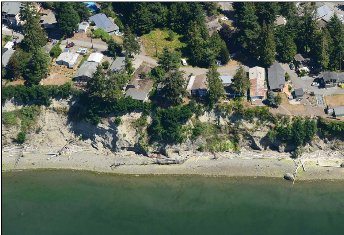
Figure 1. Hermosa Point is elevated land extending into the Port Susan forming the north point for Tulalip Bay. Fetch extends to Mukilteo nearly 8 miles away. The bluff to the north is rapidly eroding because of exposure to high energy waves, undercutting homes. This process will intensify with climate related storm intensification and sea level rise.
