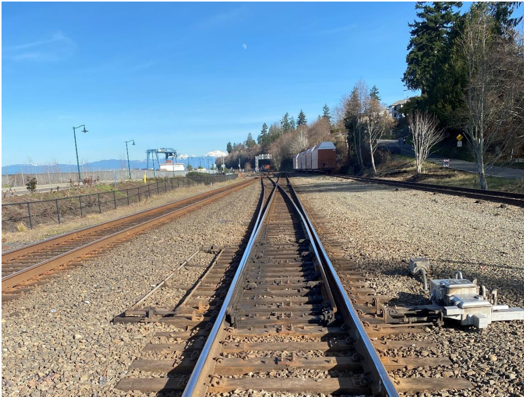
Figure 17. Three BNSF Tracks at Japanese Gulch Creek Crossing Location
