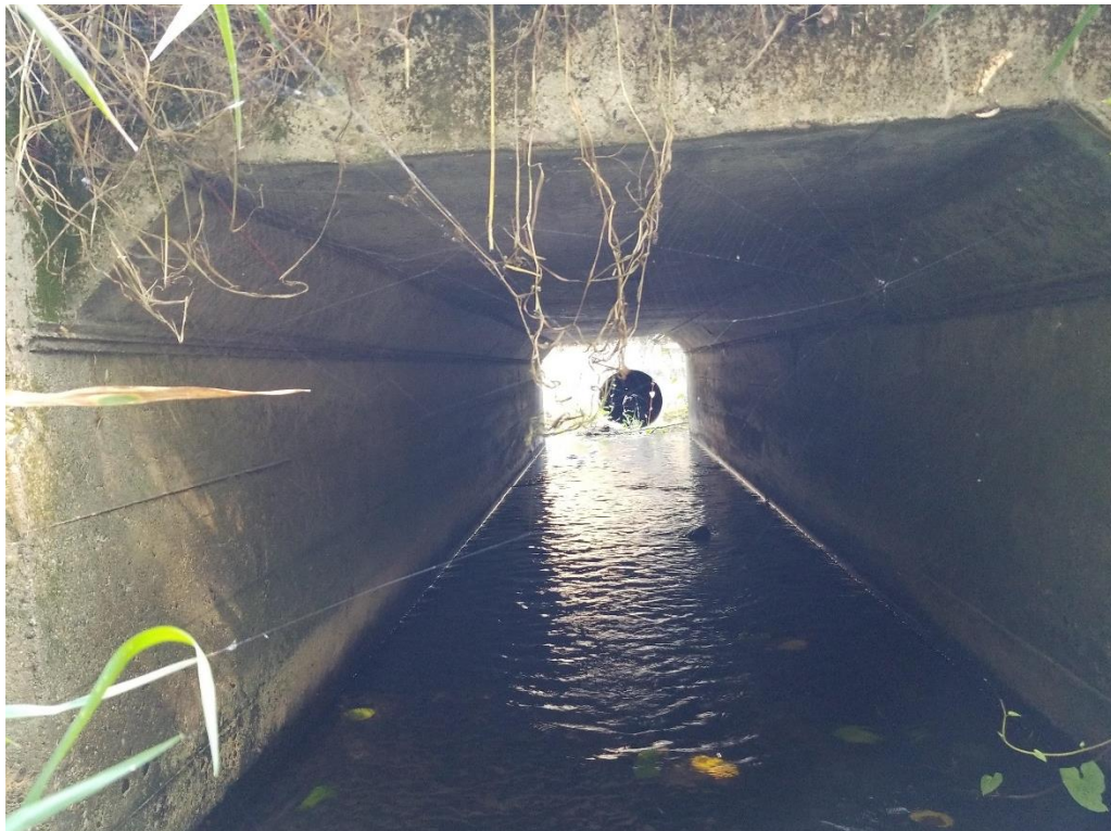
Figure 18. Japanese Gulch Creek Culvert Under Mukilteo Lane
