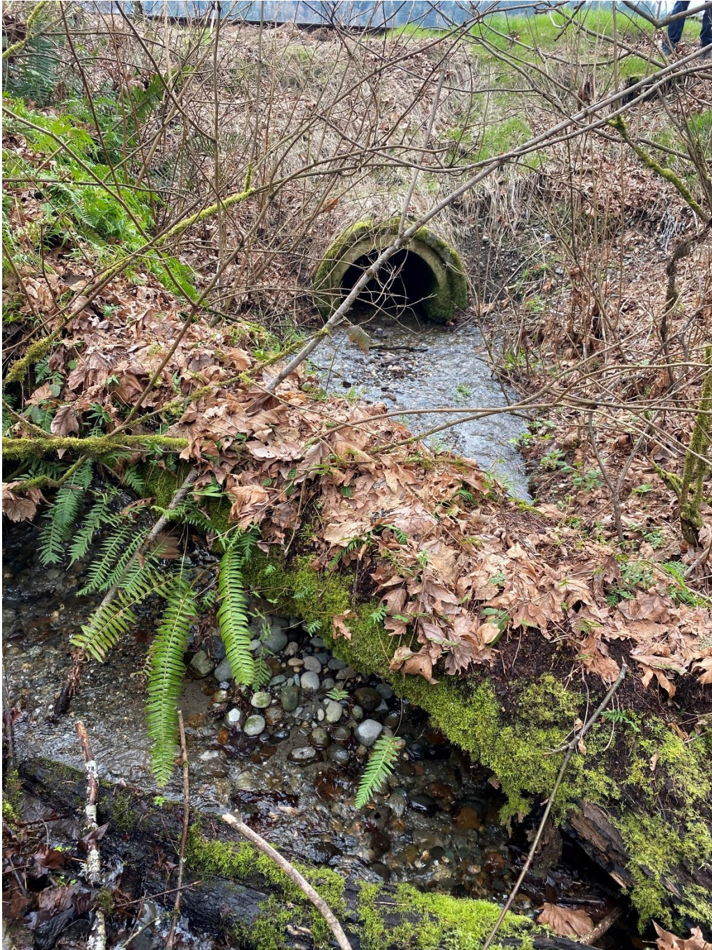
Figure 25. Unnamed Creek Channel and Culvert Inlet
