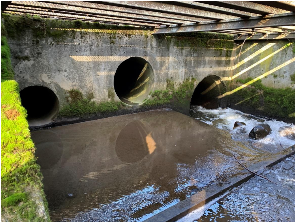
Figure 19. Headwall Upstream of Railroad Crossing
