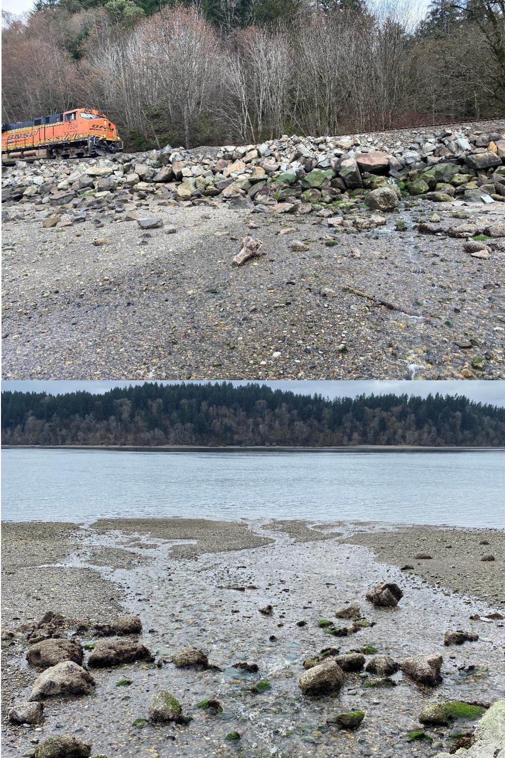
Figure 24. Culvert Outlet of Unnamed Creek
