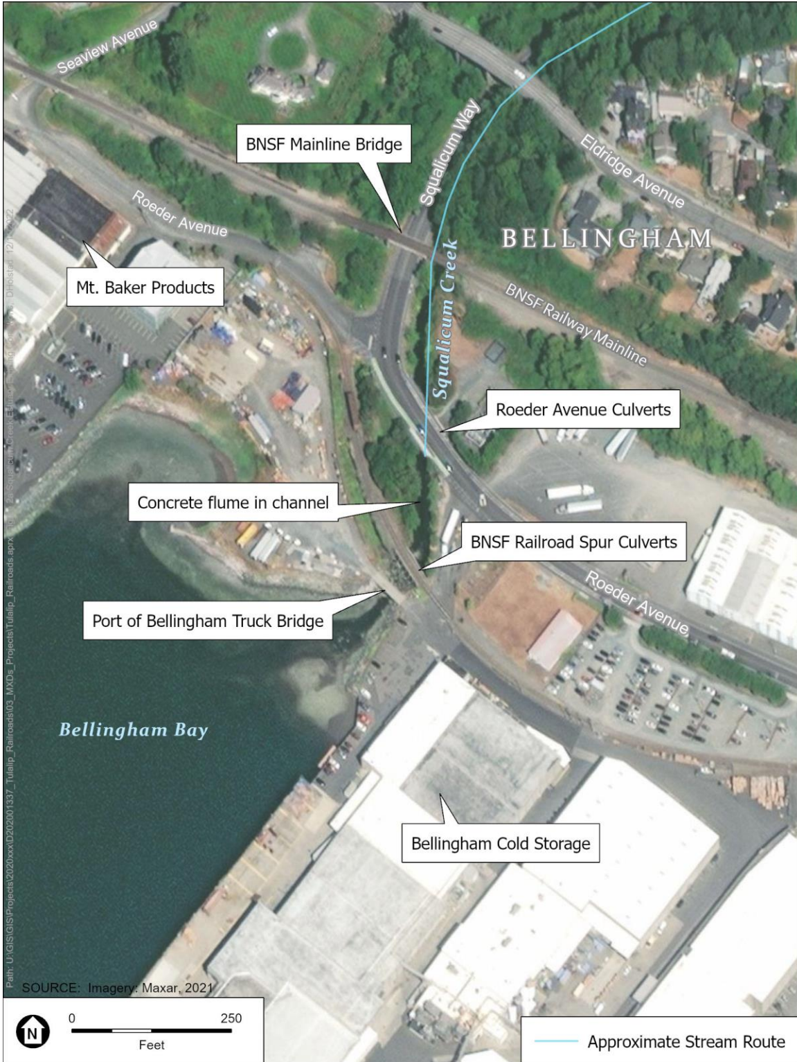
Figure 7. Squalicum Creek Estuary Site with Three Crossings
