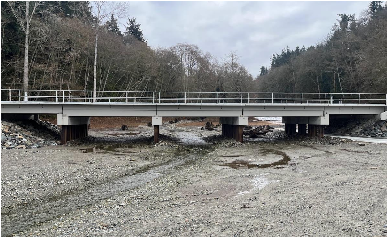
Figure 4. Railroad Crossing at Meadowdale Beach Park
