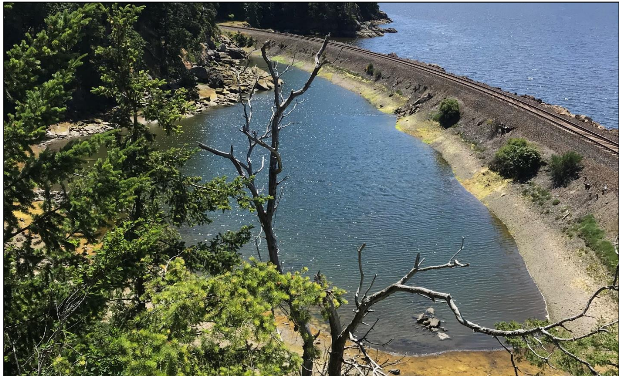
Figure 2. Historic railroad trestle south of Bellingham, WA (top; note visible openings in the railroad line running over the water) and current railroad embankment (bottom)
