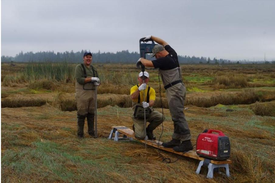
Figure 3.2. Driving stainless steel benchmark rods through the soil profile. Typical refusal depth in Snohomish installation in 2013 was approximately 18 meters.
