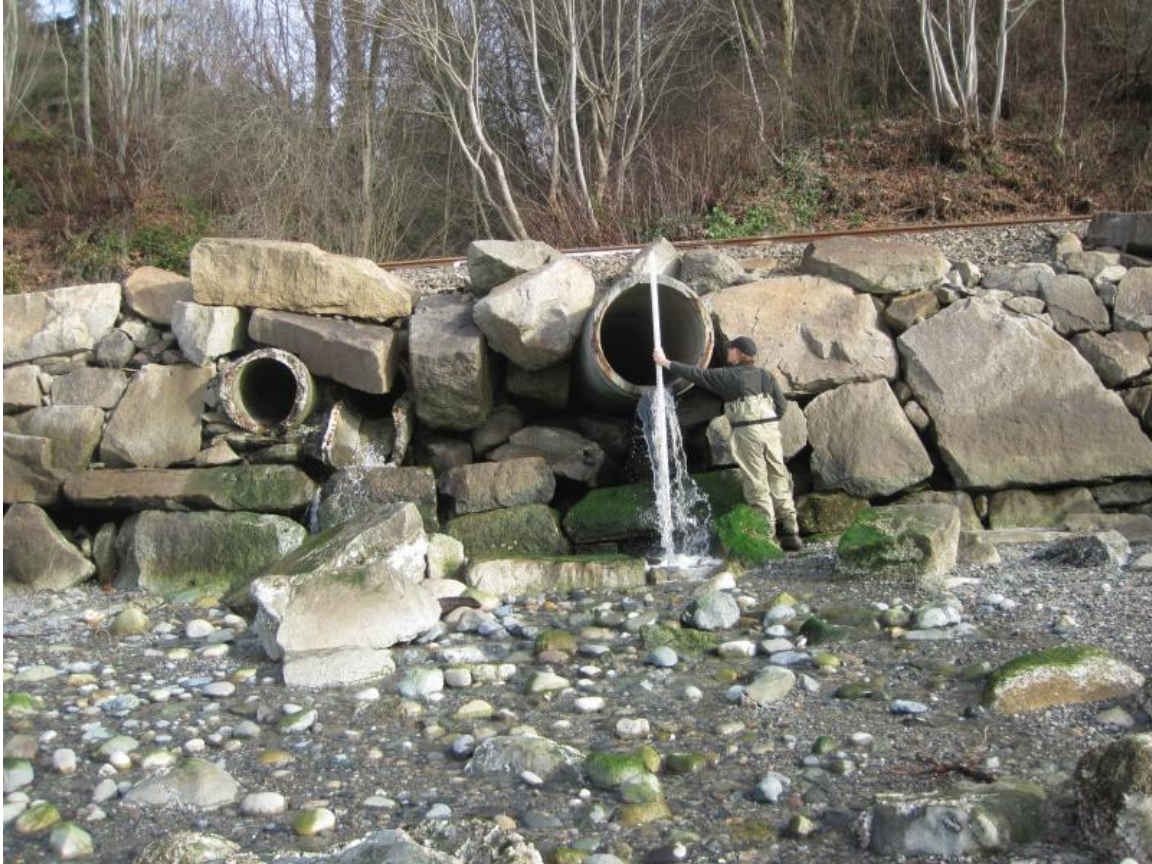
Figure 5. Example of culvert that does not backwater by tide with outlet higher than MHHW (Unnamed stream in Mukilteo, stream #54).
