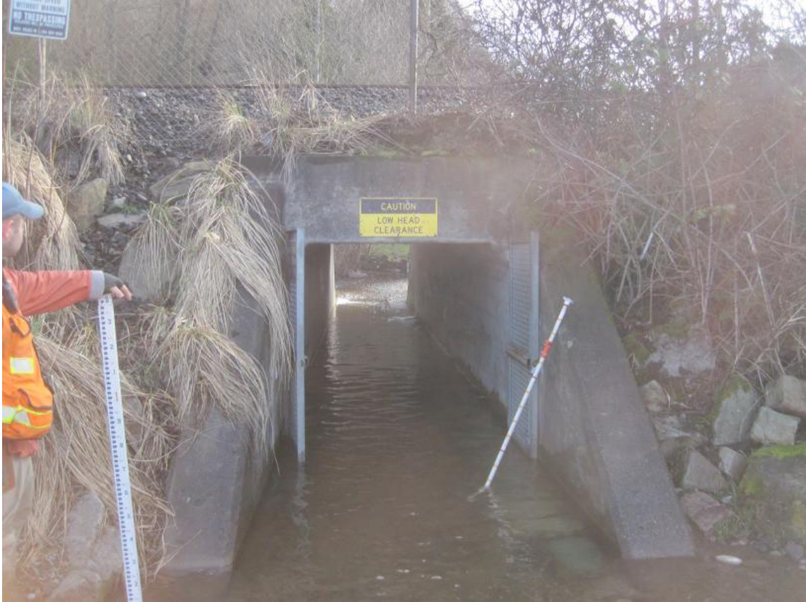
Figure 3. Example of culvert that backwaters by tide with outlet in the upper intertidal (Lunds Gulch Creek, stream #62).
