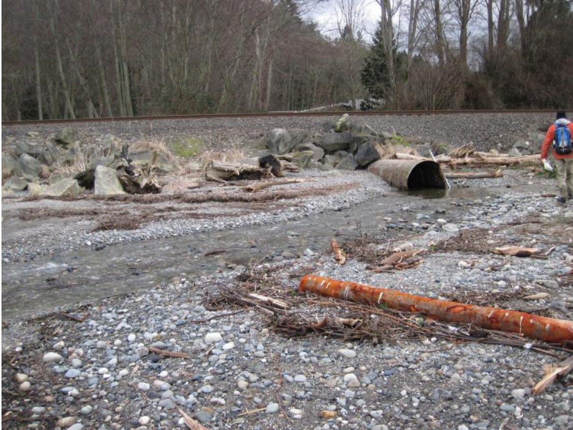
Figure 2. Example of culvert that backwaters by tide with outlet in the upper intertidal (Big Gulch Creek, stream #57).
