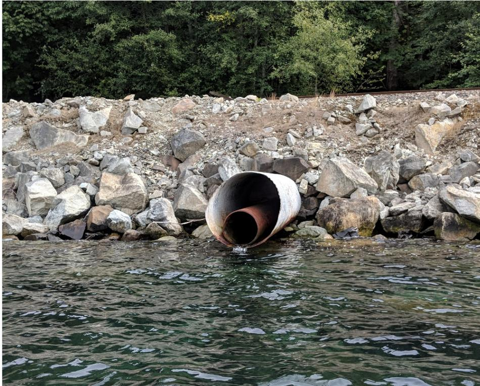
**Figure 7. Example of culvert that has been slip-lined to extend serviceable life, which has reduced the culvert size**
