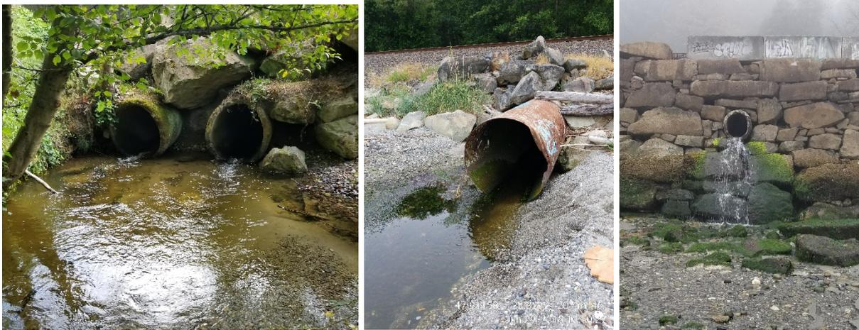
**Figure 4. Examples of round culverts encountered in field survey—dual concrete (left), metal (center), concrete (right)**
