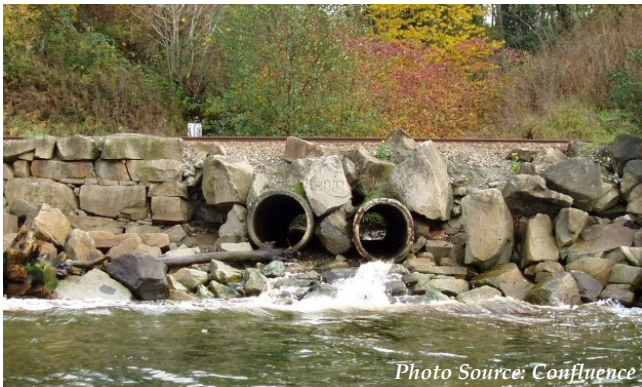
Two perched culverts conveying a small coastal stream through the shoreline railroad embankment
