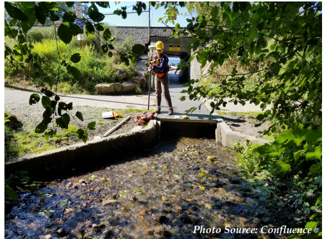
Example of a wider stream funneled into a box culvert crossing through the shoreline railroad embankment
