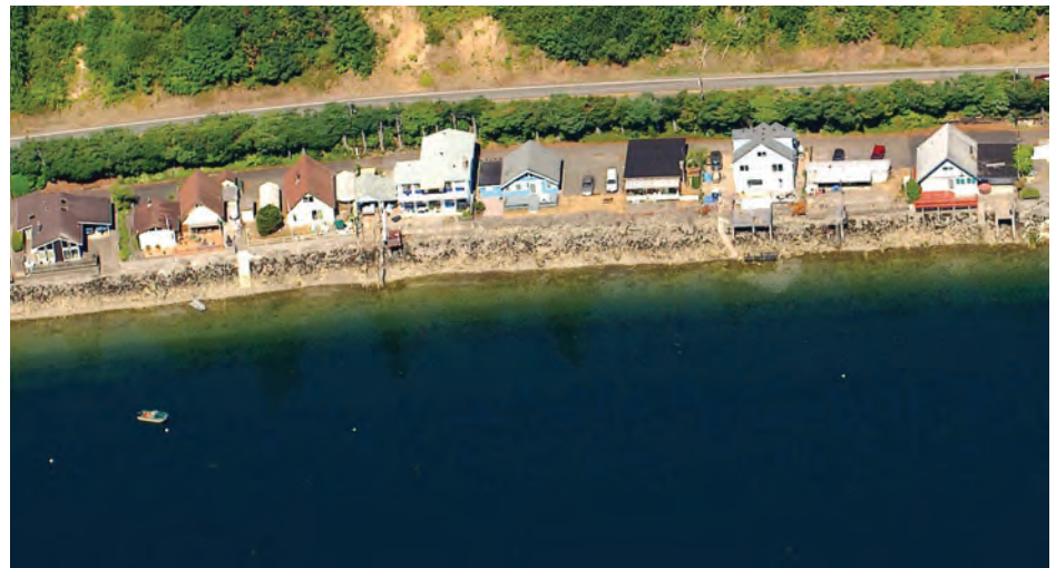
Example of shoreline armoring in the Hood Canal Watershed.
