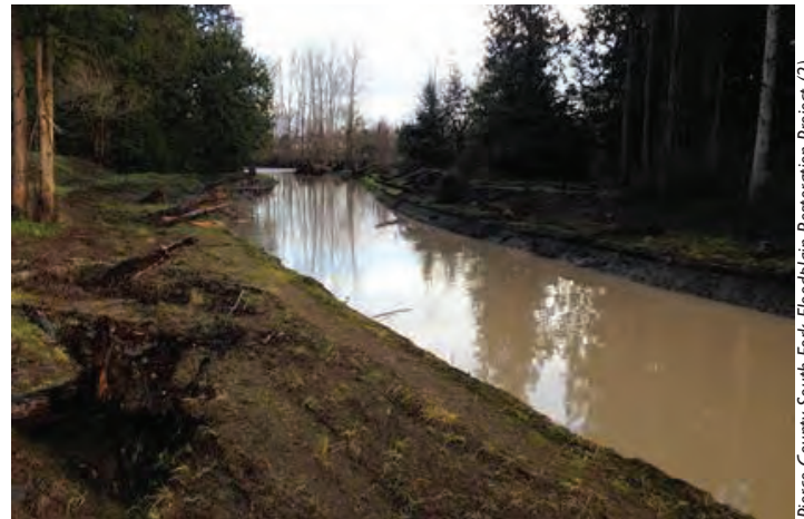
Completed South Fork Phase I Channel.
