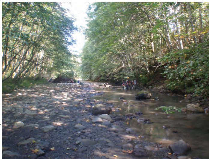
Morse Creek channelized reach through WDFW property prior to restoration, summer 2010.
