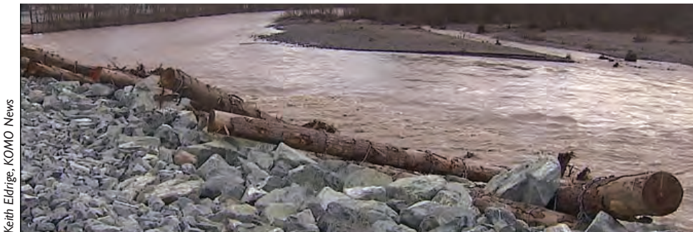
Calistoga Levee Project: This project will open up an approximately 1.5-mile-long corridor reconnecting the Puyallup River to a large portion of its historic floodplain while helping to reduce flooding and provide off-channel habitat for a range of fish species at various life stages.
