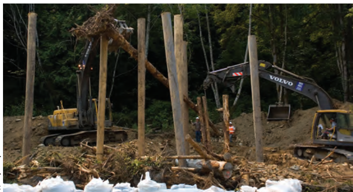
Logjam installation on Morse Creek
