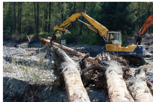
A crew installs an engineered logjam on a former tree farm acquired by the Stillaguamish Tribe.
