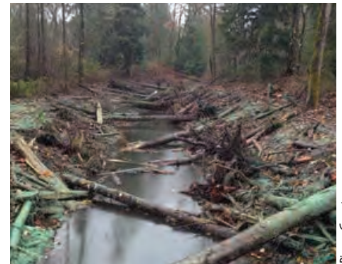
Neadham Road Levee Project: This project on the Puyallup River included the installation of 650 lineal feet of setback levee and three engineered logjams offering new habitat opportunities to local salmon populations.
