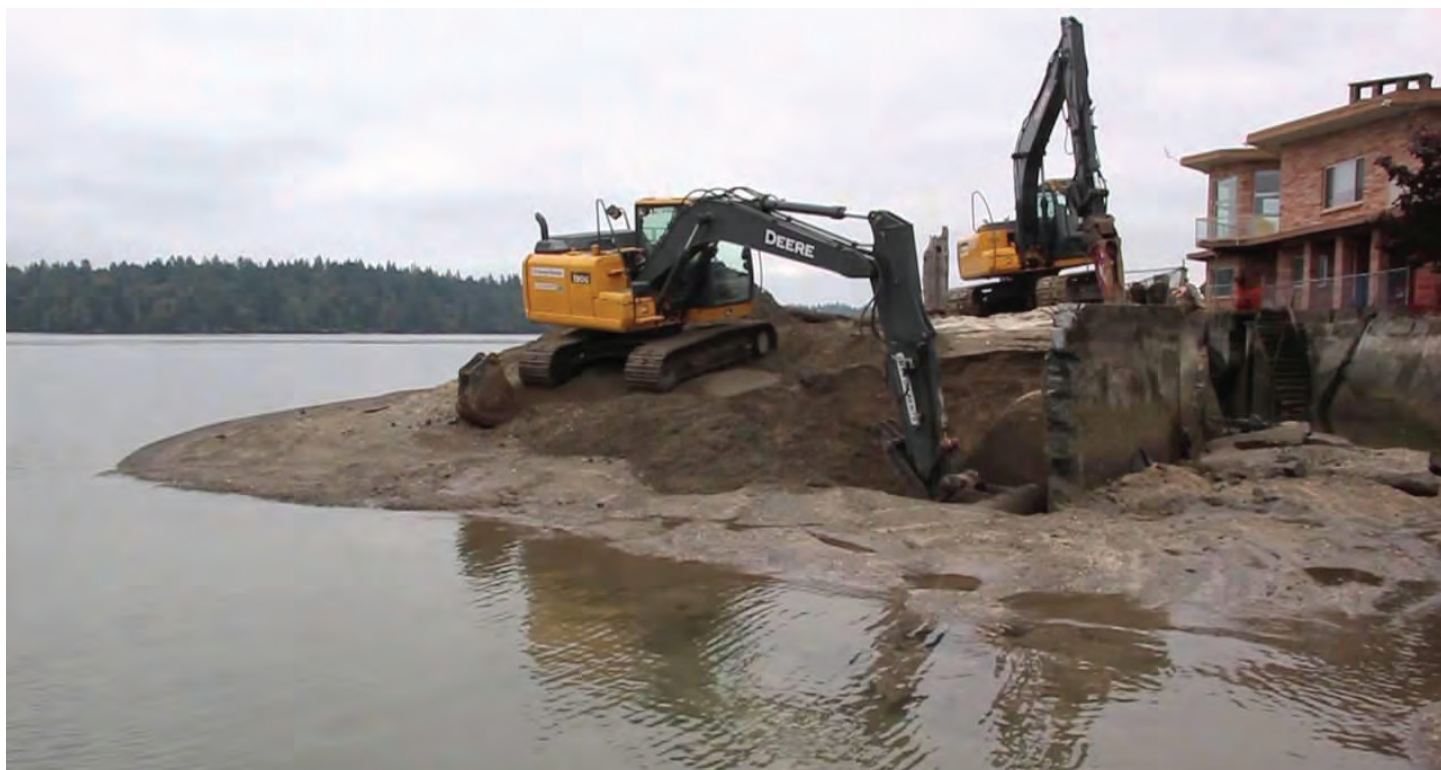
A crew removes a concrete boat basin and ramp.
