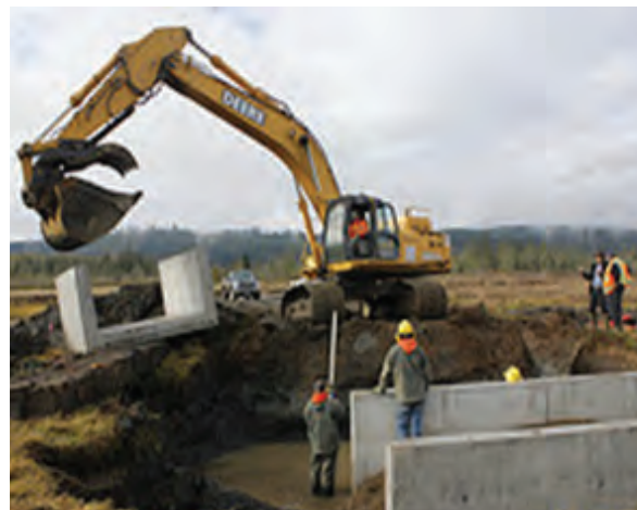
Dirt is moved and land is surveyed for the proper placement of a box culvert in the Skokomish estuary.
