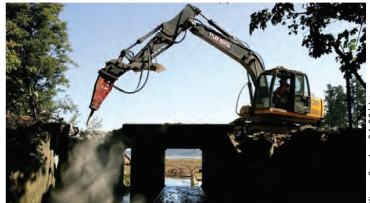
Workers pulverize Kittyhawk culvert.
