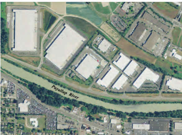
Example of impervious surface near the Puyallup River.
