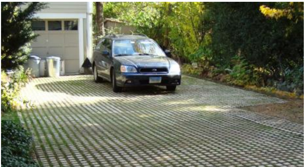
Porous Paver Driveway (Soil Retention)
