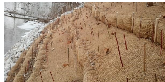
Newly planted bank with dogwood stakes
