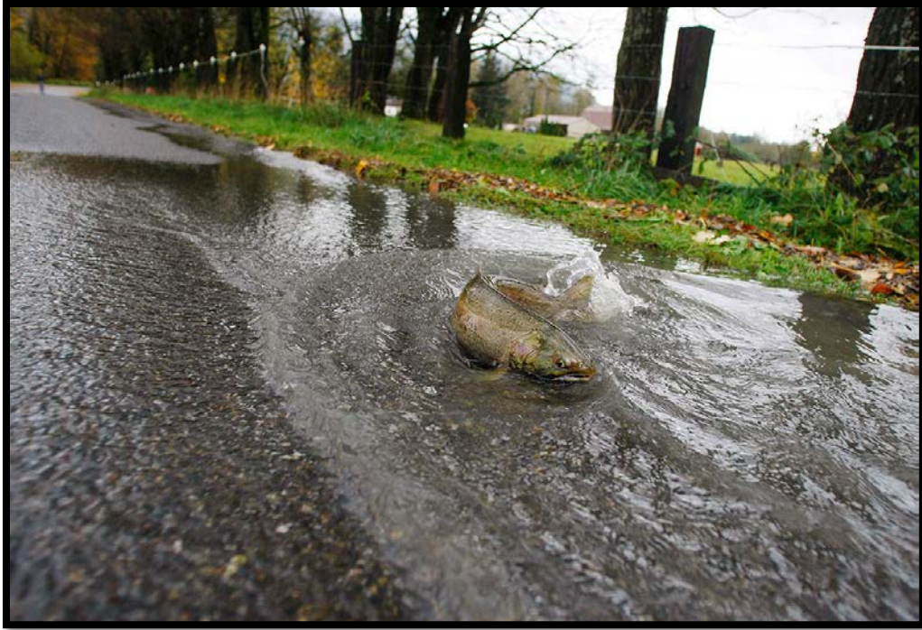
A salmon attempts to swim over the roadbed of 399th Street outside Gold Bar in October, 2009, after waters from the Wallace River flowed over the road during flooding. (Mark Mulligan/Herald file photo; https://www.heraldnet.com/opinion/editorial-no-avoiding-duty-to-restore-salmon-habitat/ )
